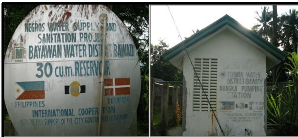
Figure 6. Nangka Pumping Station and 30 cu. m. Reservoir
